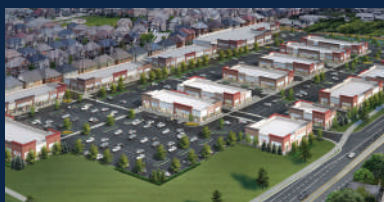
MAYFIELD COMMERCIAL CENTRE
